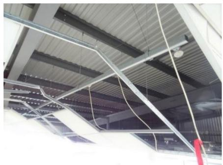
Plate 4.4: Roof structure visible through area of damaged ceiling
