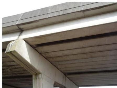
Plate 4.9: Expansion gaps between concrete panels
